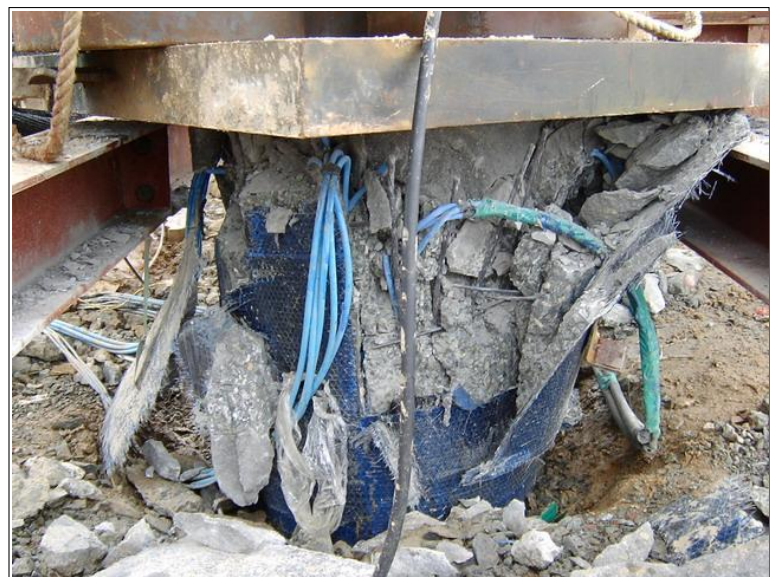
Fig. 1 The pile head immediately after the break
